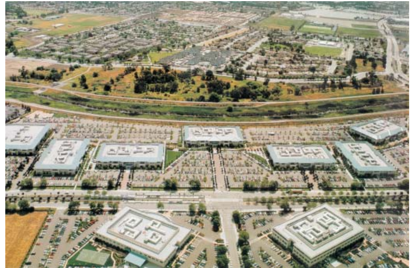
Typical Silicon Valley corporate campus swims in a sea of parking while being segregated from residential, commercial, and open space areas. Robert Cameron, 1998. Above San Francisco, Cameron and Company
