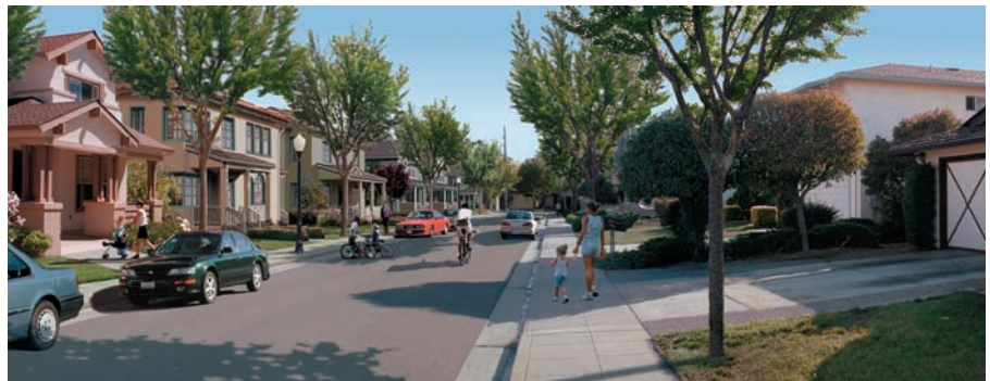
Before and after: Infill can transform neighborhoods in a way that enhances their character.
