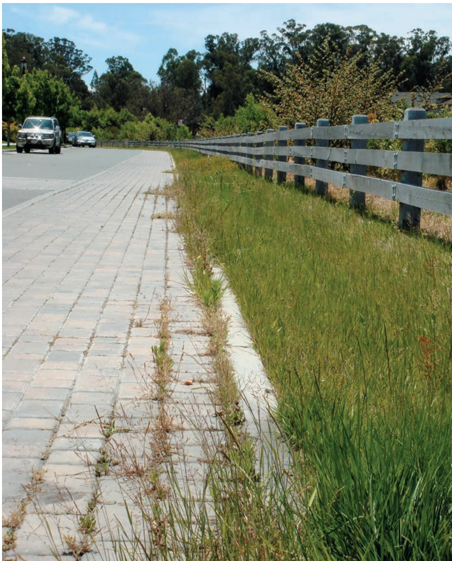
Curbless streets and swales are design strategies that treat stormwater as a resource rather than a waste product. Permeable paving without curbs allows rain to flow into the ground before going to the Bay, cleaning the water and reducing flood risk.
