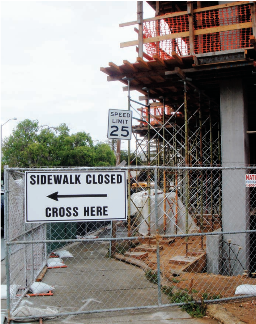
Cities can ease the construction process by making it less costly to temporarily close sidewalks or streets and by providing police support and timely inspections.
