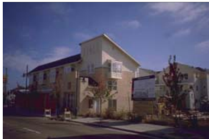
Live-Work Lofts San Pablo Ave, Emeryville Live-work units and townhouses.
