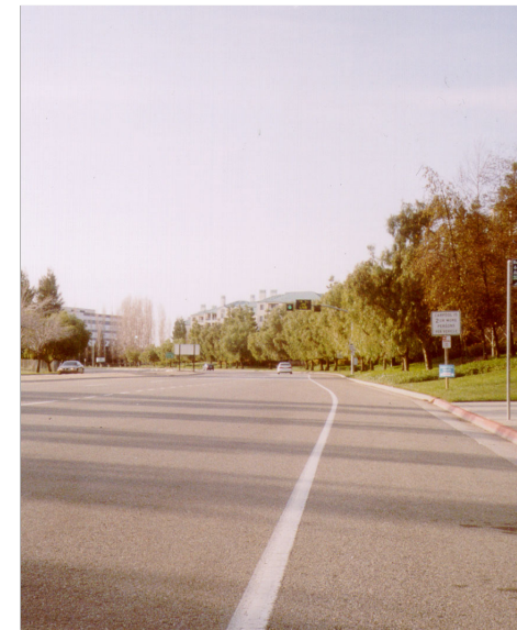
Montague Expressway, San Jose
