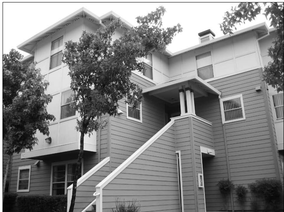
Creating more housing options, like these apartments in Fairfield developed by the Solano Affordable Housing Foundation and Mid-Peninsula Housing Coalition, will help balance Solano County's housing market
